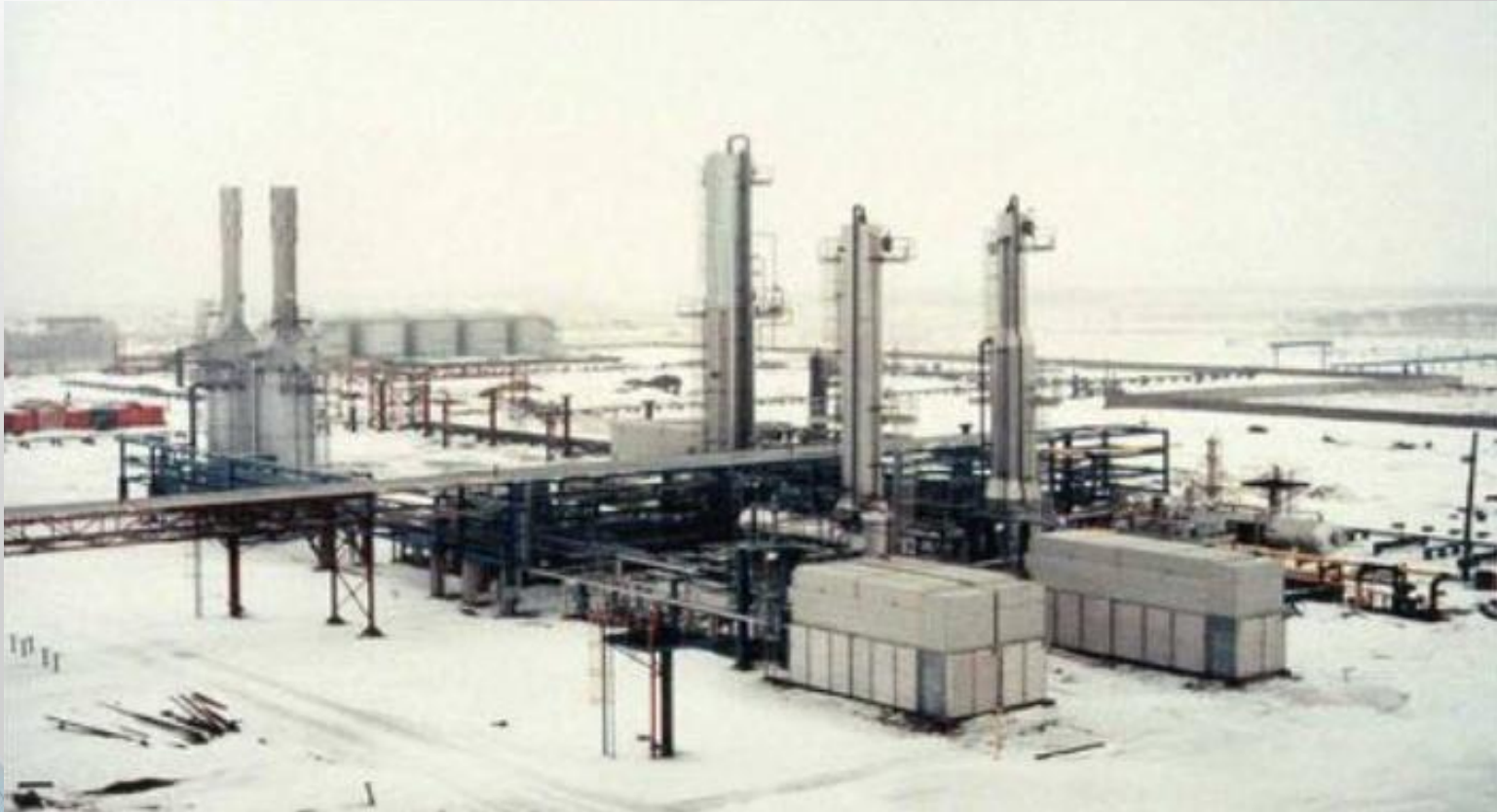
11,000 BPD Modular Refinery. Kazakhstan. PROPAK
