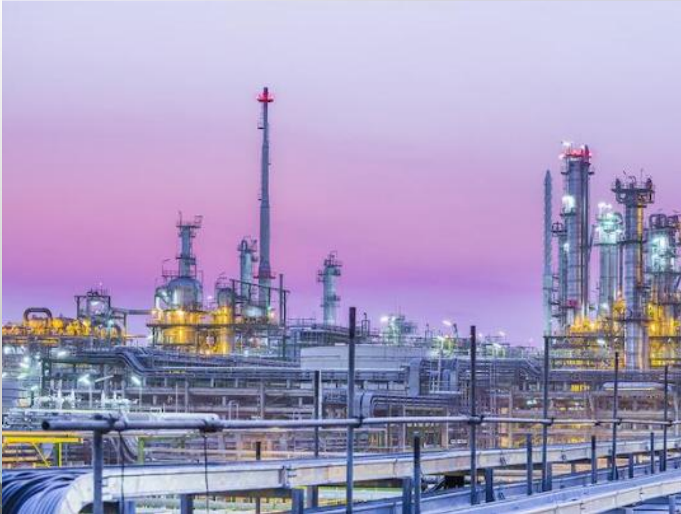
Cabinda Refinery – Angola - 30.000 bpd. VFuels
