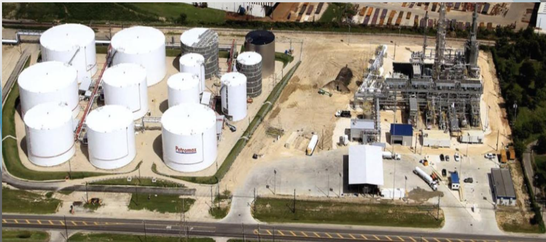
PETROMAX Modular Refinery 25,000 BPD. Houston TX. Basic Equipment
